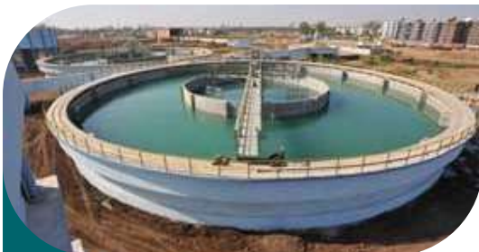
Intake well of a TTP within Surat's Industrial Water Supply Initiative. Source: Surat Municipal Corporation (n.d.).
