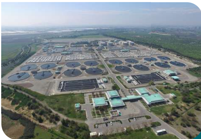
Aerial view of the La Farfana biofactory Source: ohstgo.cl (n.d.).
