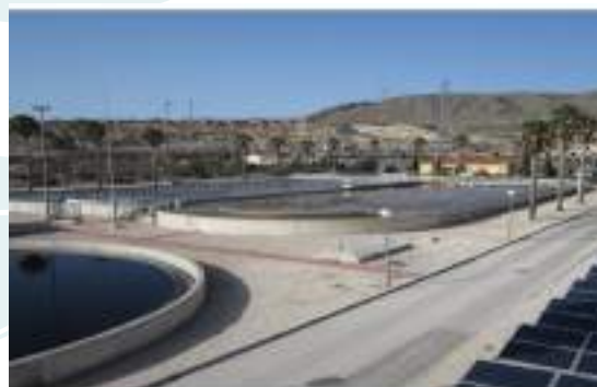
Cieza sewage treatment plant in Murcia, where water is reclaimed for irrigation. Source: Gomez Espin et al. (2025)
