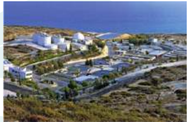
View of the Limassol – Amathus water reuse system (Cyprus). Source: Maffetone et Gawlik 2022
