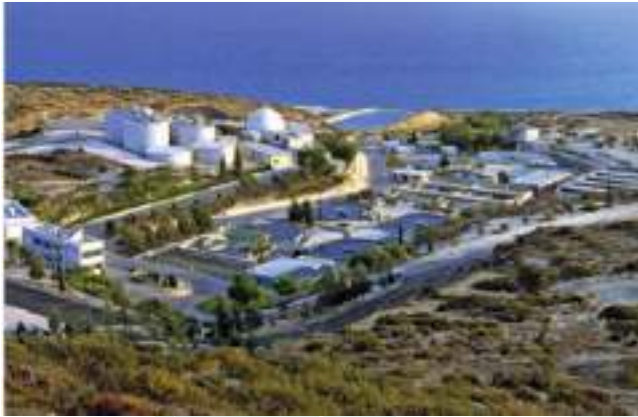
View of the Limassol – Amathus water reuse system (Cyprus). Source: Maffettone et Gawlik 2022
